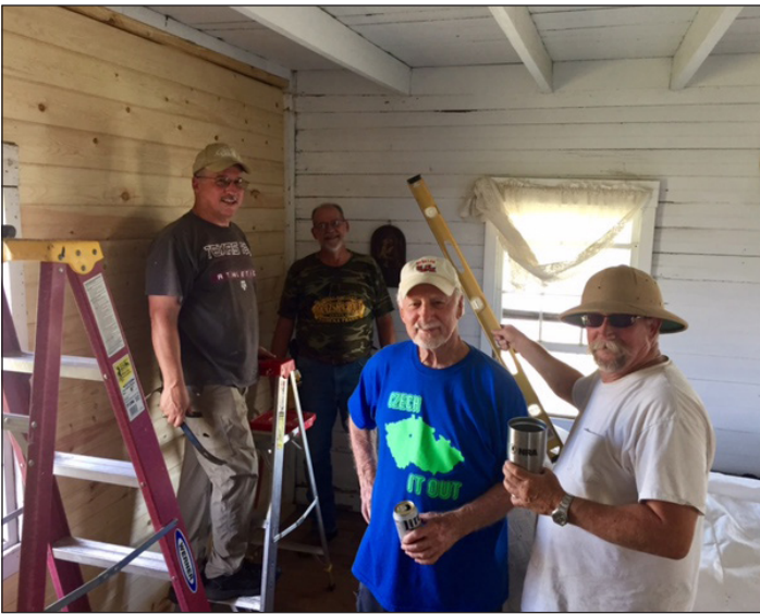
Mark Jašek, Art Migl, Jim Jašek, and Thomas Motal replaced an interior wall in the Migl House that had been damaged by Hurricane Harvey.
